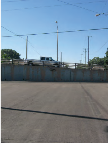
View of the Clark Street viaduct looking south along Pine Street.
