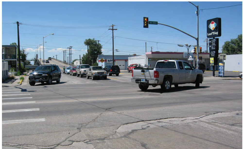
Clark Street Viaduct - Eastside Looking West
