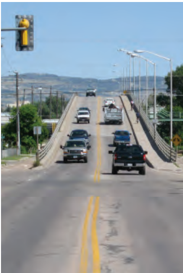
Clark Street Viaduct - Westside (Looking East)
