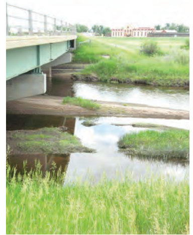
Laramie River Bridge upstream looking west.
