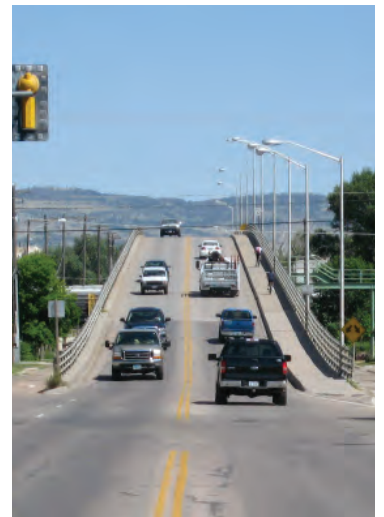
Clark Street Viaduct - West Side Looking East
