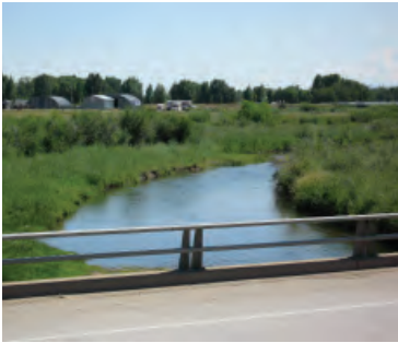
Laramie River Bridge looking upstream.
