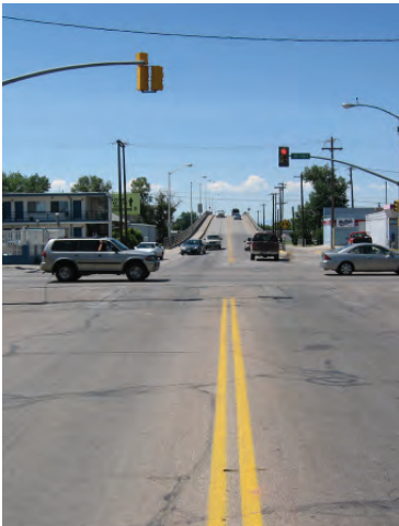
View of the Clark Street viaduct looking west.
