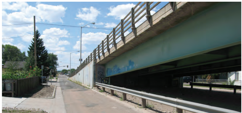
Service Road Adjacent to Clark Street Viaduct (Looking West)
