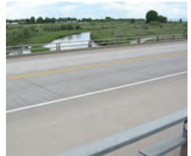
Laramie River Bridge looking upstream.
