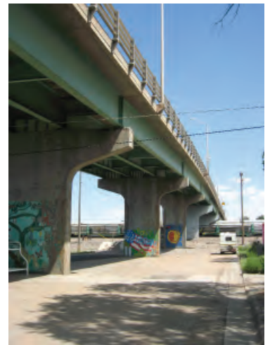
Clark Street Viaduct
