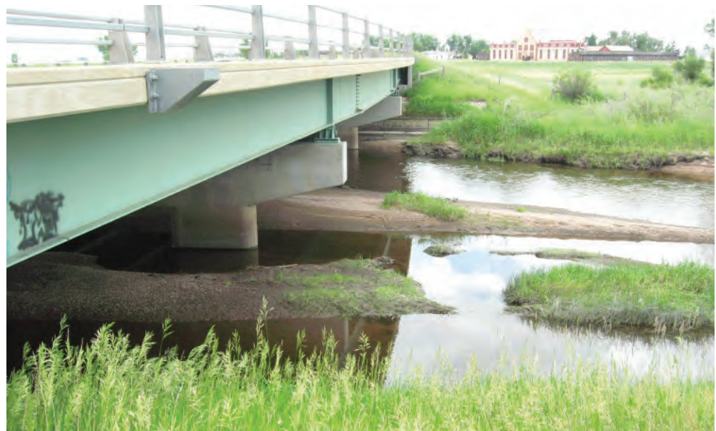
Laramie River Bridge (Looking West)
