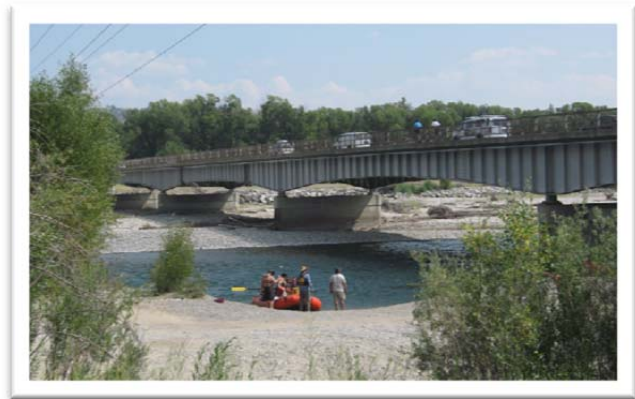
Recreationists near the WYO 22 Snake River bridge.
