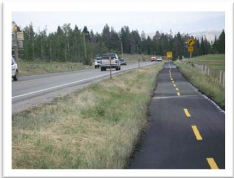
Existing bike path along WYO 22
