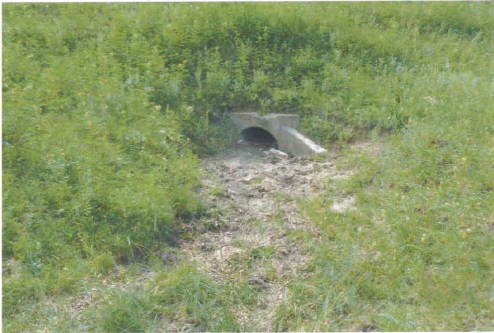
Photo 3: Culvert outlet along WUS-2.
