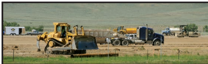
Work on the runway and taxi extension at the Pinedale Airport.
