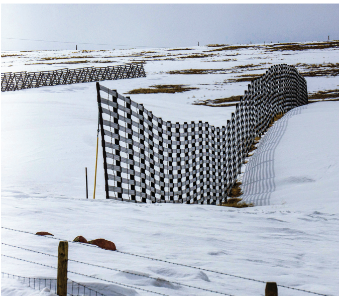
Snow fence controls the most serious drifting in areas along Wyoming's highway system.
