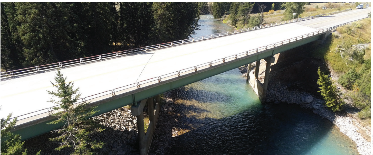
Wyoming's state highway system includes nearly 2,000 bridges that WYDOT maintains.
