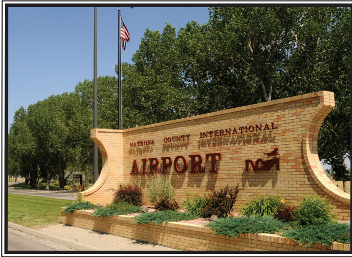
Many projects were completed in 2011, including improvements at the Natrona County International Airport.
