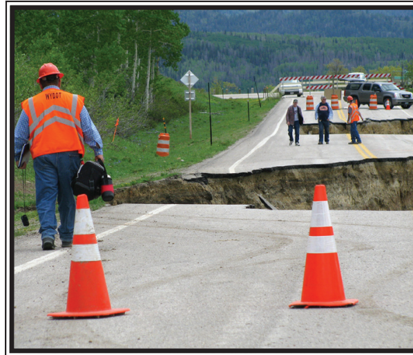
Damage from flooding and landslides have been a major concern for the Engineering & Planning Division.
