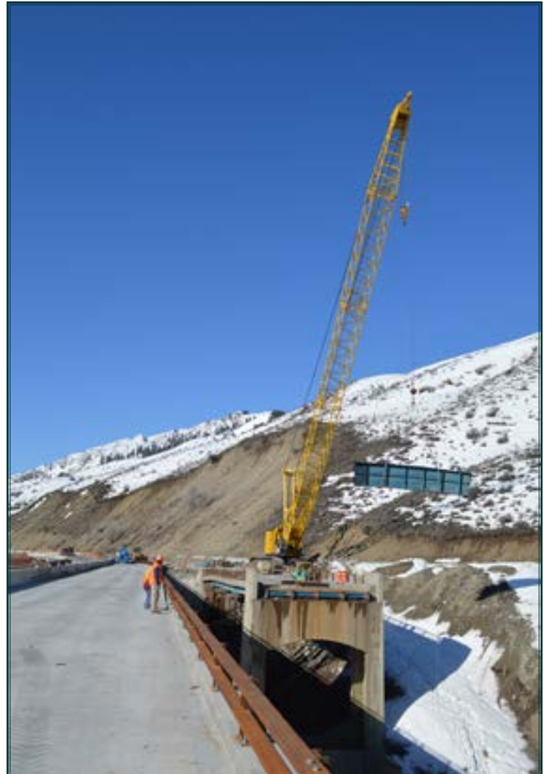
Steel removal progresses on the old Hoback Junction bridge.
