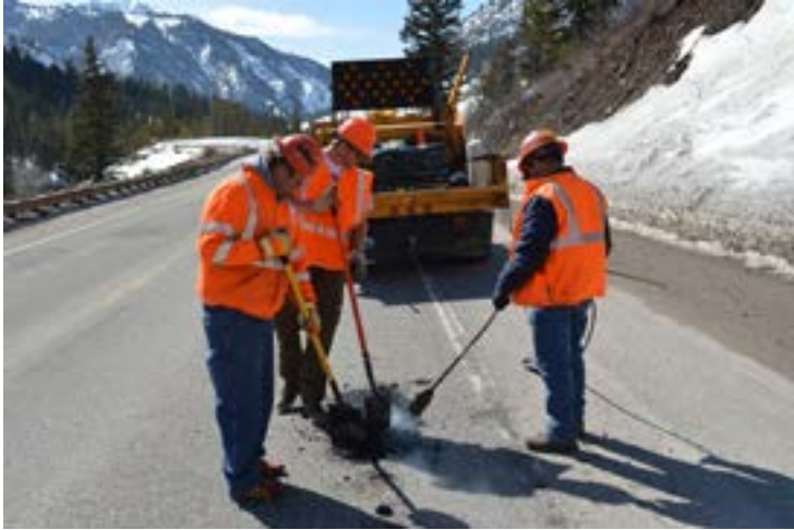
Pothole patching, US 26-89.
