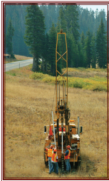
The Geology Program completed 742 holes for a total of 17,672 lineal feet of drilling for subsurface investigations.
