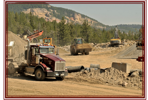
Work continued in 2012 on US 16 between Worland and Buffalo.
