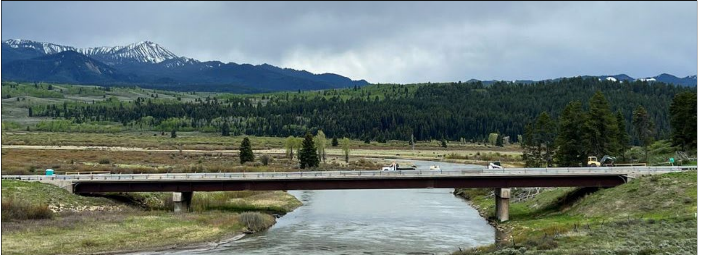
Buffalo Fork of the Snake River bridge on US26/287 in Teton County
