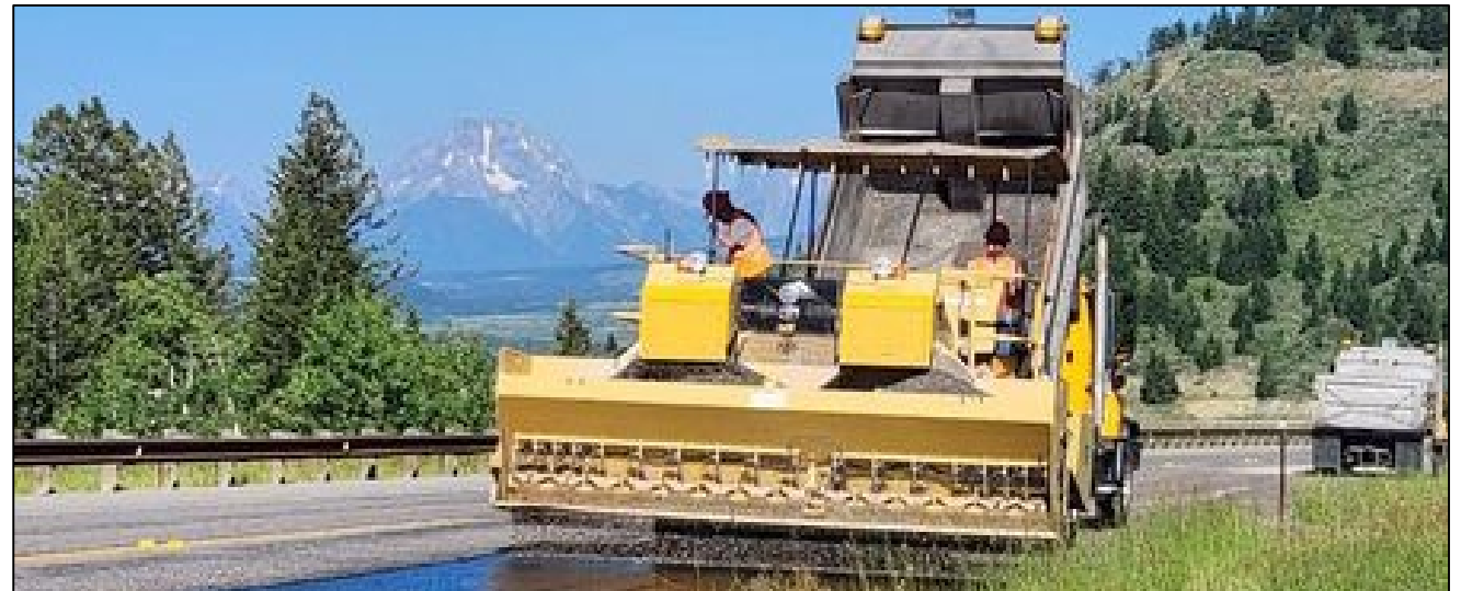
Maintenance chip sealing on US26/287 over Togwotee Pass, 2023
