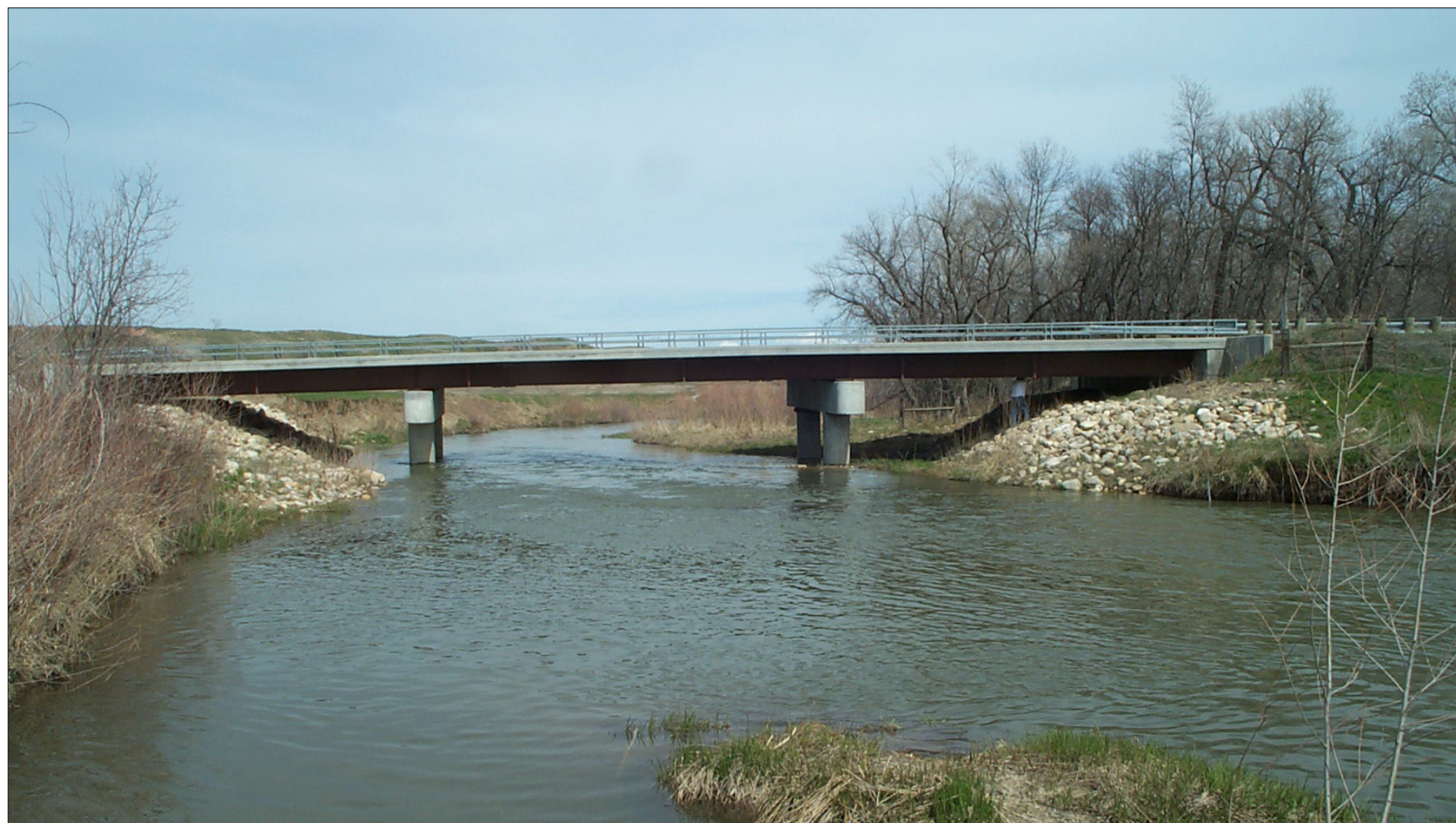
Bridge on WY 338 over the Tongue River
