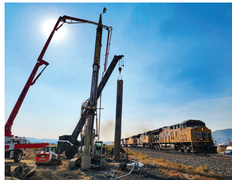
WYDOT is in the process of drilling 48-foot shafts at the project location.
