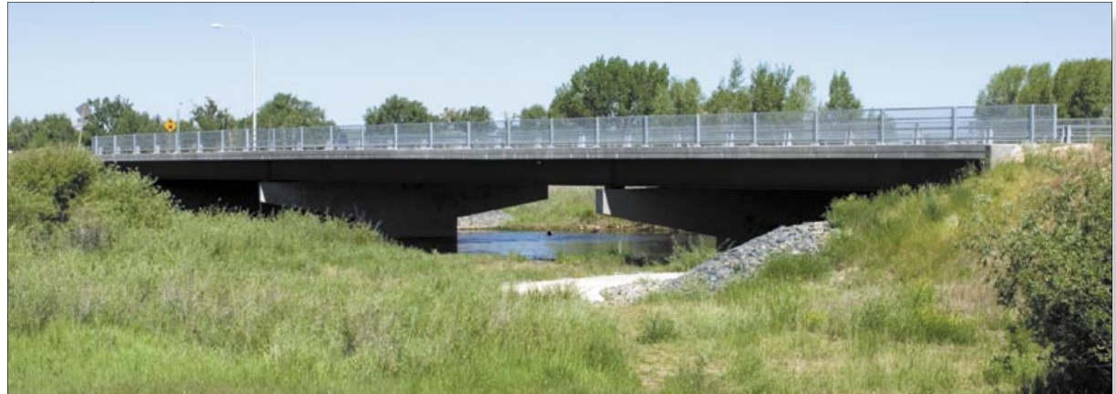
Garfield Street / Big Laramie River bridge replacement, Laramie. Photography by Horse Creek Studio
