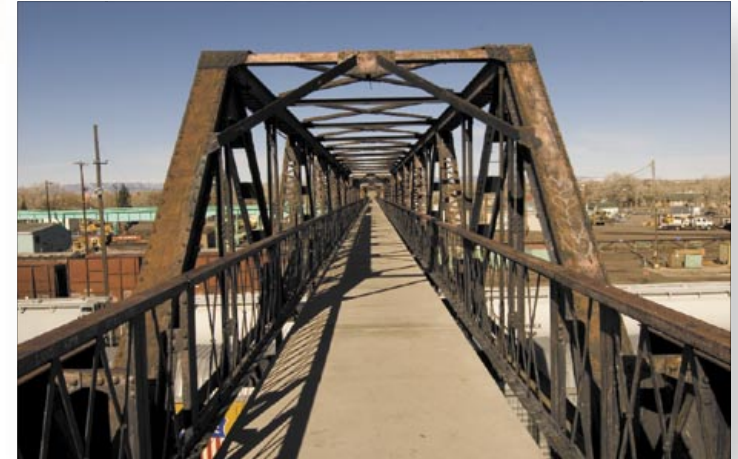
Historic Downtown Laramie footbridge maintenance project. Photography by Horse Creek Studio
