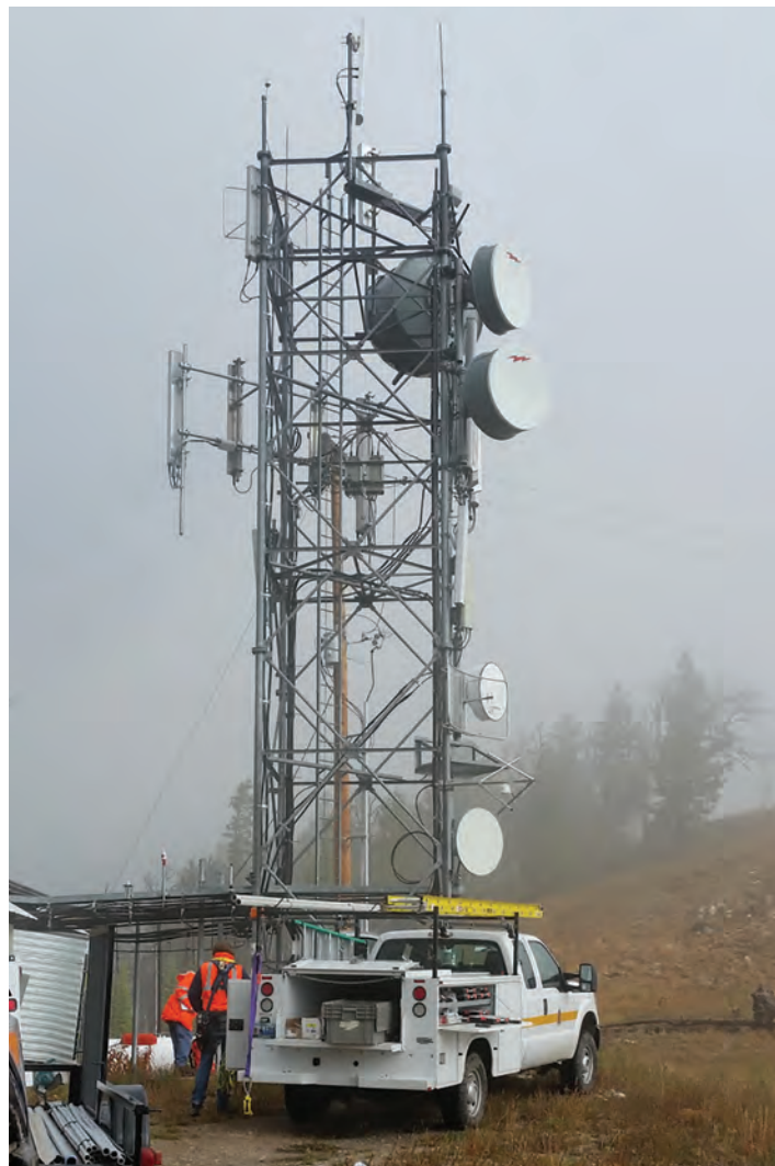
The Teton Pass radio tower.
