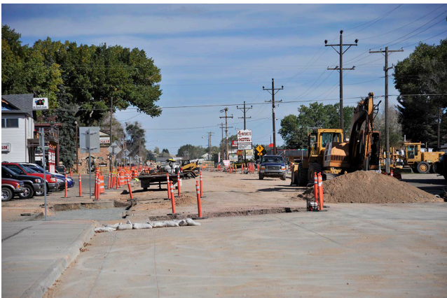
Douglas fuel tax project under construction.
