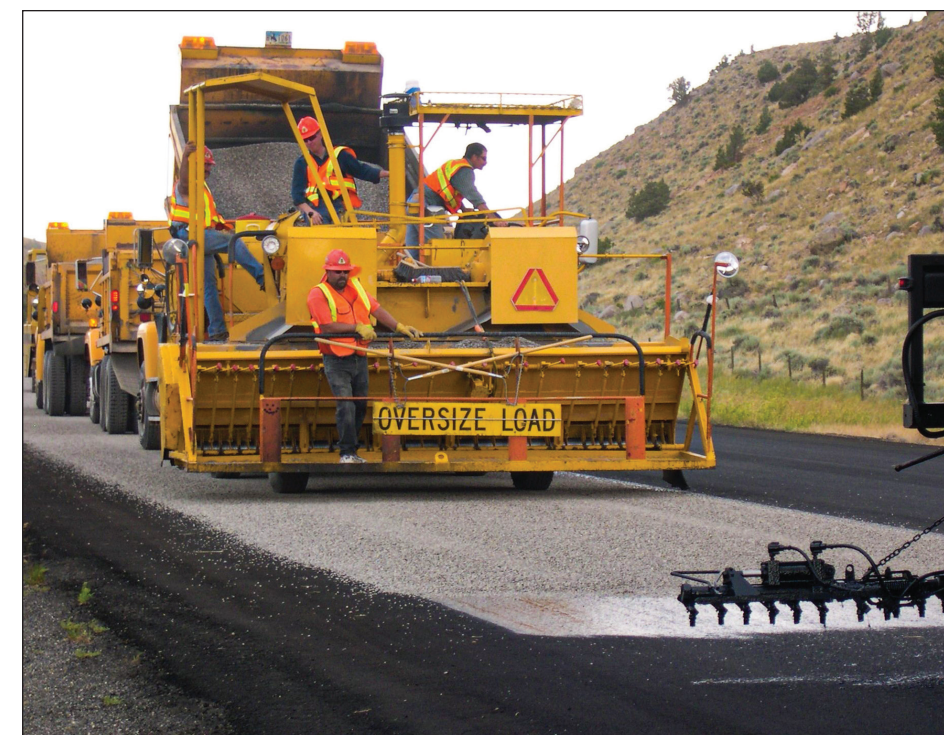
A WYDOT District 5 crew applying chip seal to the newly paved asphalt.
