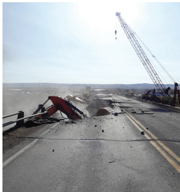
Crews with Reiman Corp. take chunks out of the Curtis Street bridge over Interstate 80 in Laramie during demolition May 16. The 60-year-old bridge had been deteriorating, causing yearly maintenance to allow live traffic.
