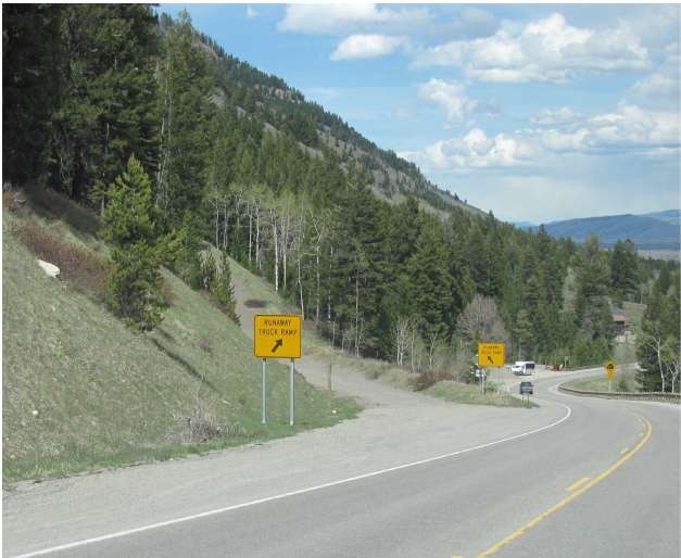
The old sandpile ramp on WYO 22, Teton Pass.
