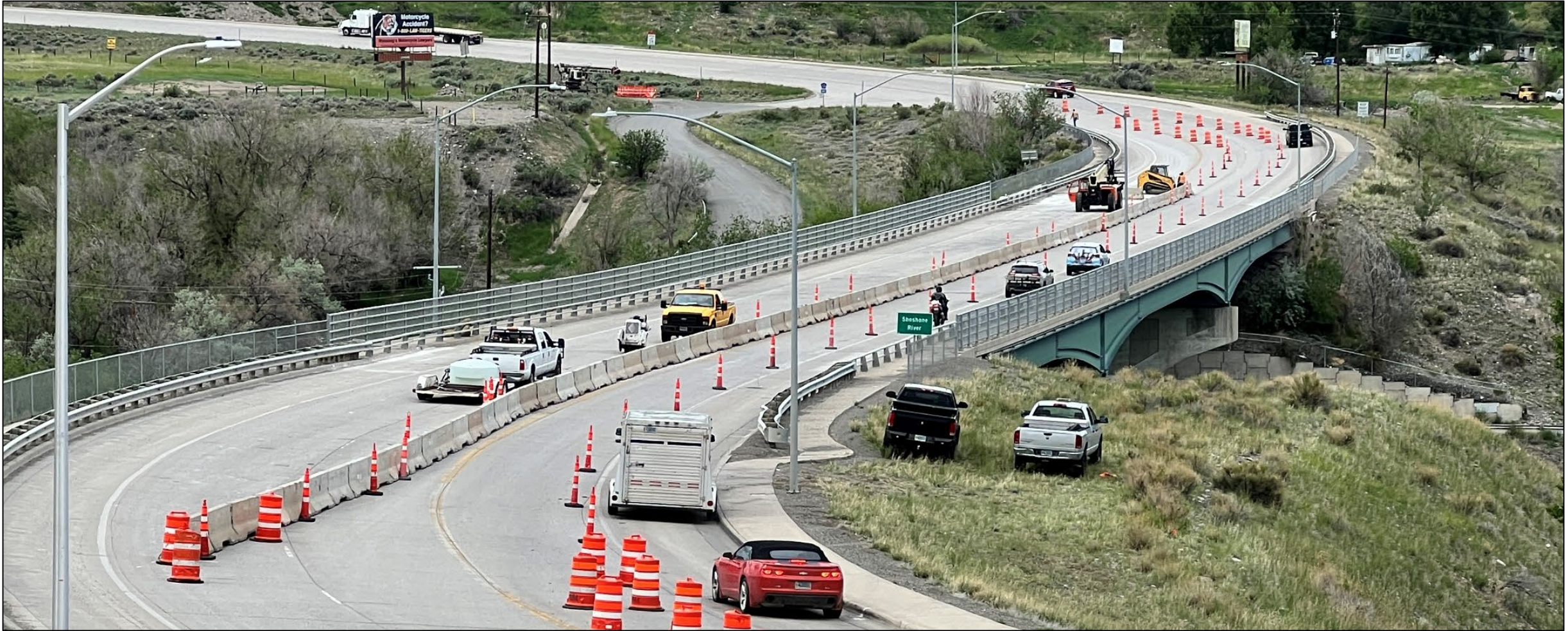
WY120 bridge rehabilitation, spring and summer 2023
