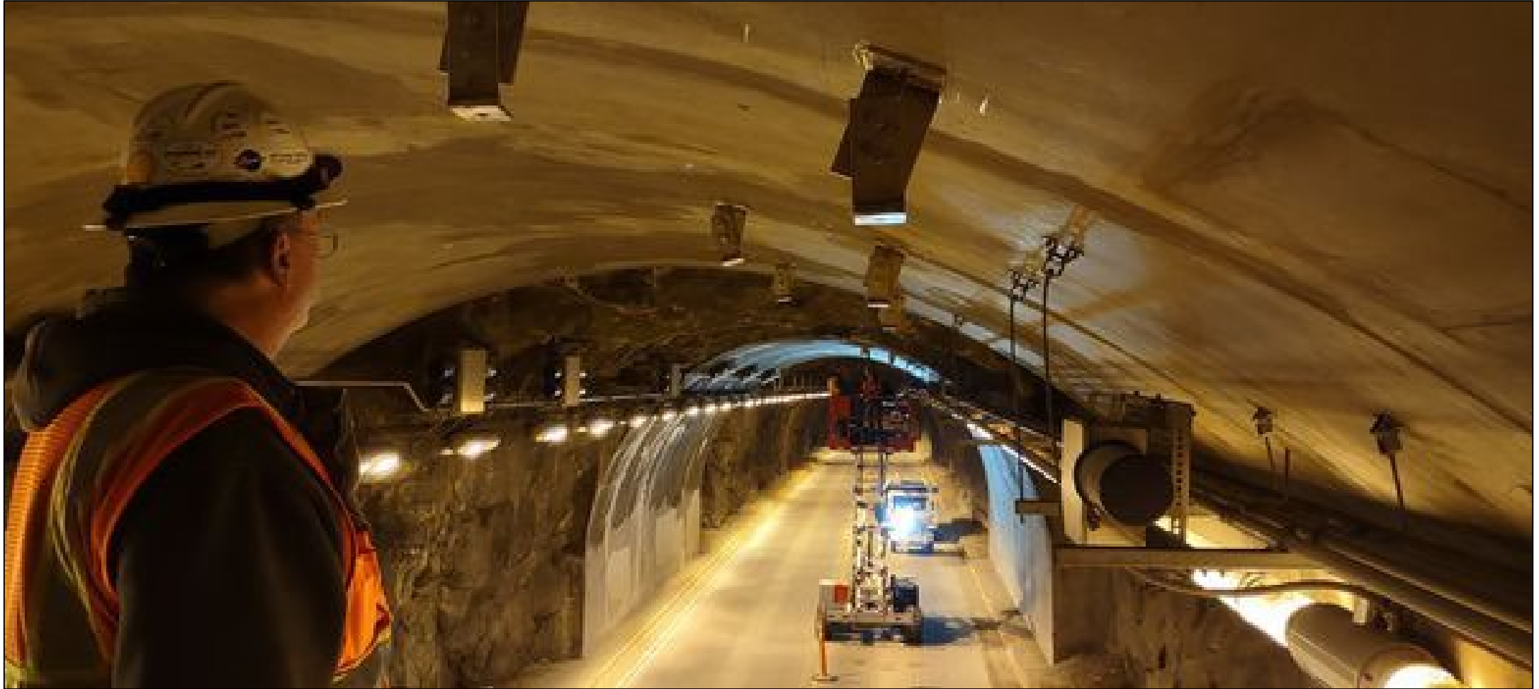
Cody tunnel lighting work, summer 2023
