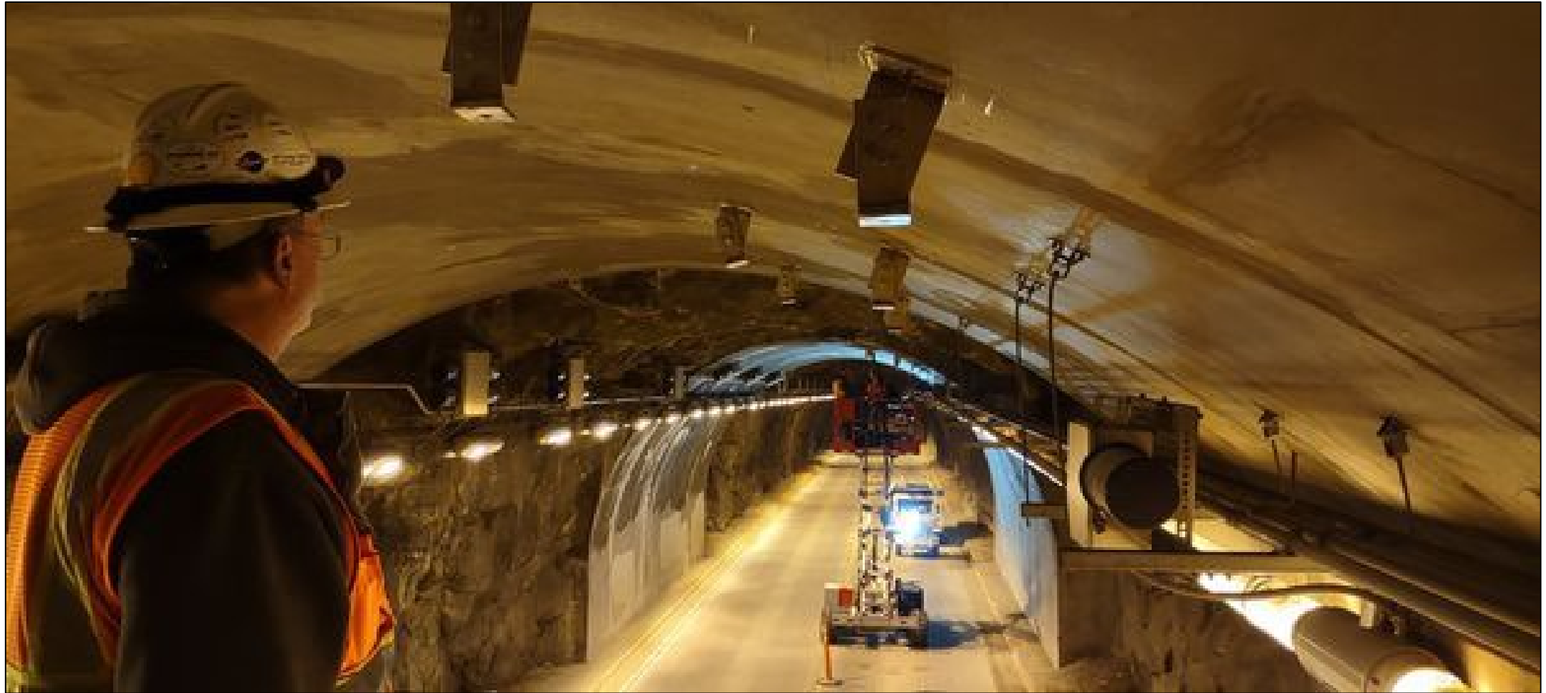
Replacing tunnel lights, U.S. 14/16/20, west of Cody, 2023
