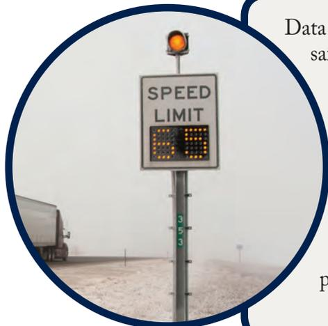
Data continues to indicate that VSLs have a significant positive impact on public safety by reducing crash totals and severity and road closure duration and frequency.
