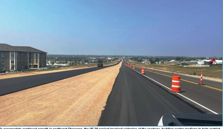
To accomodate continued growth in northeast Cheyenne, the US 30 project involved widening of the roadway, building center medians to help restrict turning movements, performing ADA upgrades and installing a new signalized intersection at Whitney Road.
