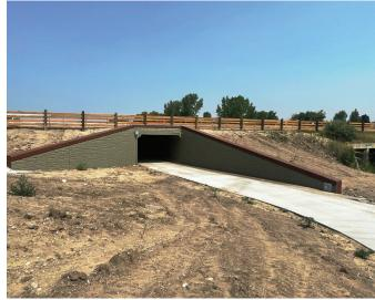
The project included replacing a culvert that was part of the city of Cheyenne's greenway trail network. The new culvert was placed just west of the old one and will fix the flooding issues the previous culvert suffered.
